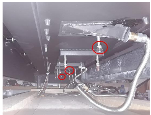
EX 2: AIR SHUTTER ADJUSTMENT UNDER YOUR FIREPLACE
