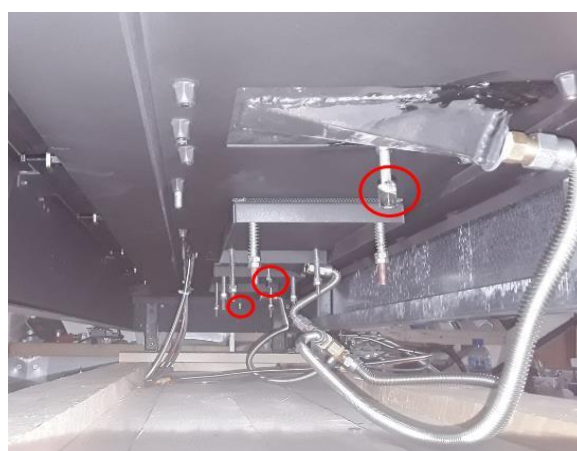
EX 2: AIR SHUTTER ADJUSTMENT UNDER YOUR FIREPLACE
