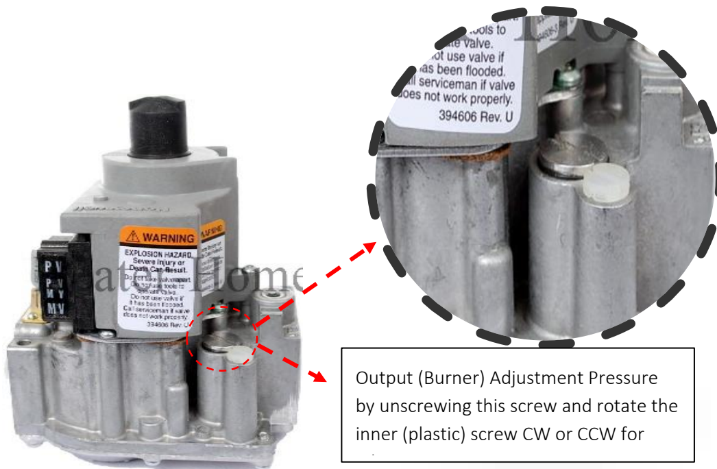
Honeywell Valve Adjustment
